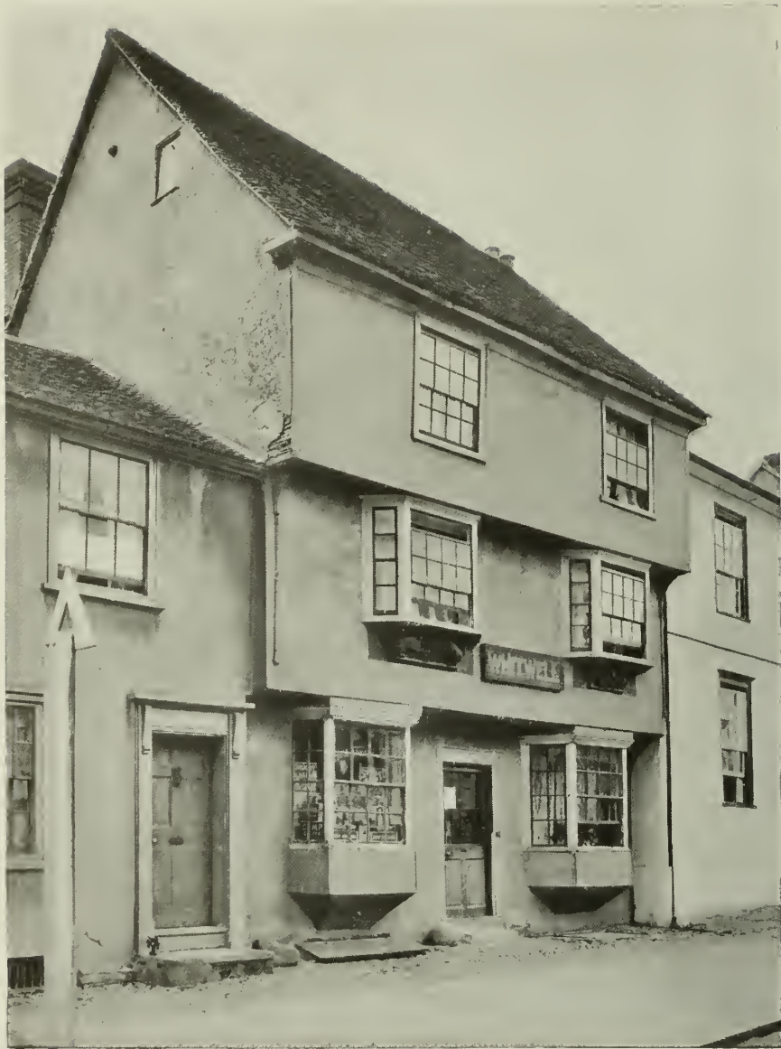
THAXTED: (15). THE RECORDER'S HOUSE, TOWN STREET. Late 15th-century.
